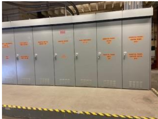
Figure 31 & 32 - NMSU Turbine and Essential Distribution Board
