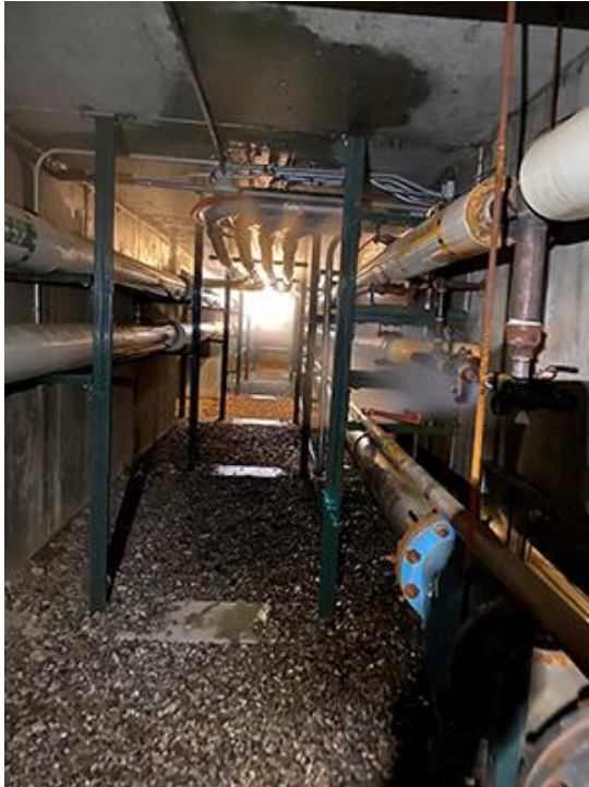
Figure 15 - Zuhl Library Tunnel; Building 461
