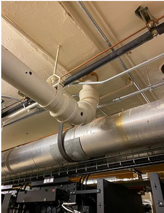
Figure 6 & 7 - Waste plumbing, from the floor above, runs through the ceiling of the Milton Hall Distribution/Data Center and terminates (with a clean-out) in front of the active Lumen rack. Also, pictured above are ceiling drains that are installed above all of the active gear.
