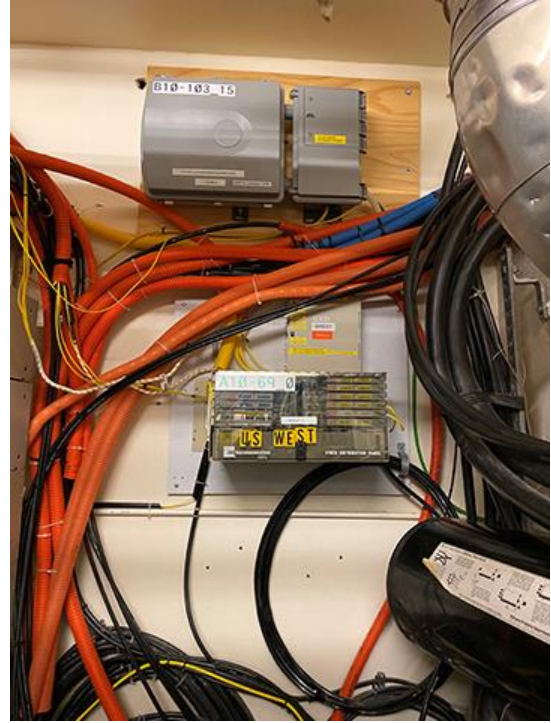
Figure 9 - Service provider MPOP (T-Mobile and Lumen)
