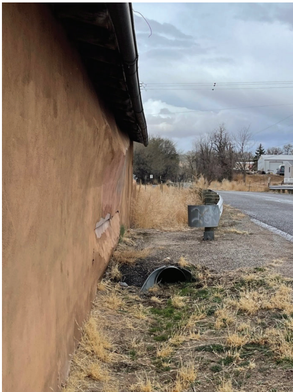
View of adobe erosion below stucco surface. This condition is typical.
