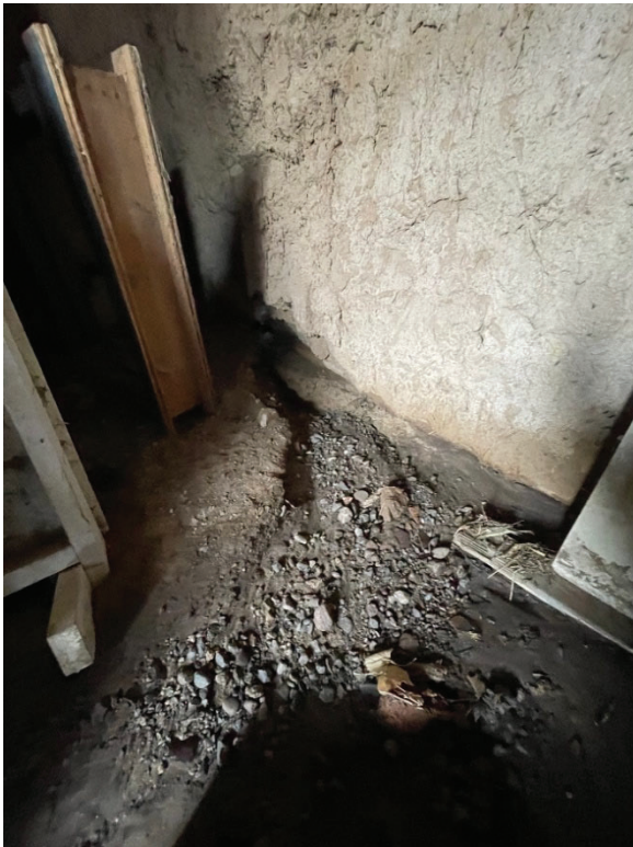
Interior view of water coming in through bottom of adobe wall eroding the base of wall and causing differential settlement.
