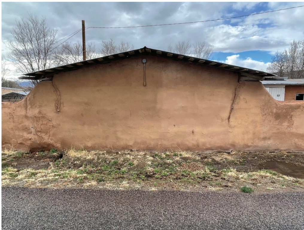
View of through-wall cracks, street runoff water infiltrating building at base of wall and differential settlement.
