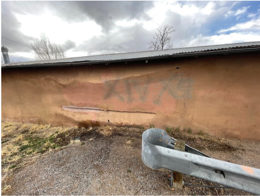
View of adobe erosion below stucco surface. This condition is typical.
