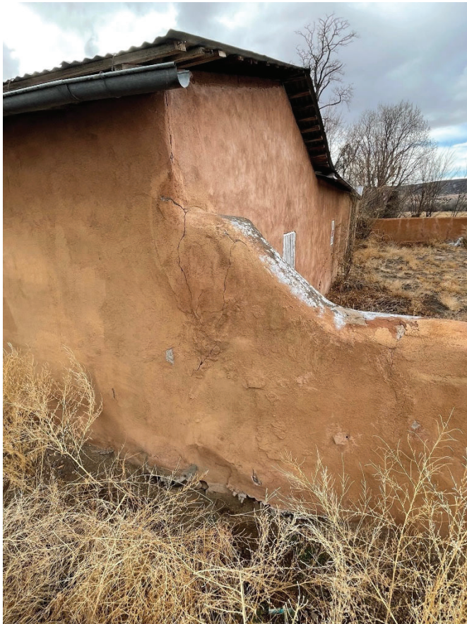
Up close view of street water runoff cutting through adobe wall and undermining the adobe foundation causing differential settlement of second building along roadway.
