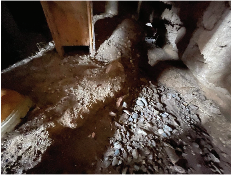
Interior view of water coming in through bottom of adobe wall eroding the base of wall.
