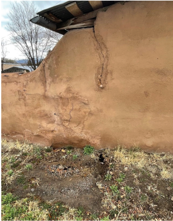
Upclose view of street water runoff cutting through adobe wall and undermining the adobe foundation causing differential settlement.
