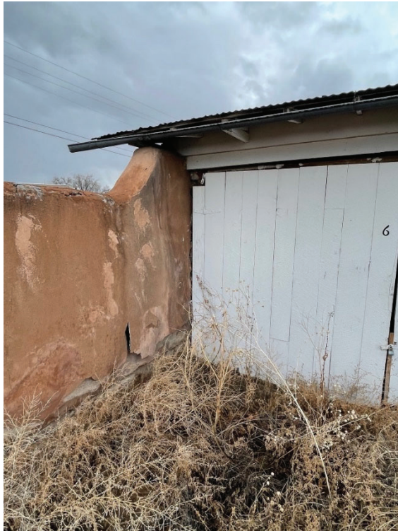
View of water damage to the adobe walls and adobe erosion below the stucco surface. This is typical.
