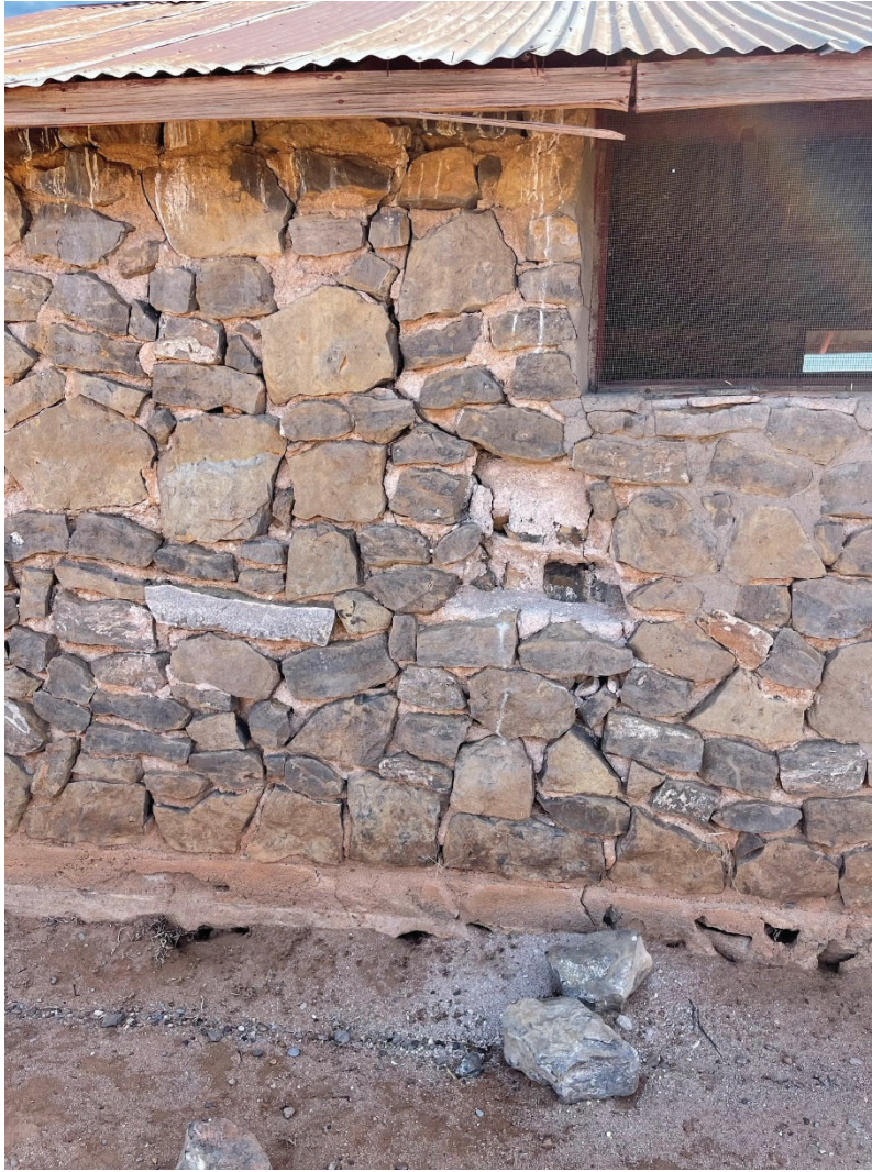
View of corner settlement, powdered setting mortar, rotted wood and rusted galvanized roof panels
