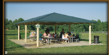
Community Sports Park, Cummings, GA: This economical design stands up to heavy use and keeps looking great. 24' x 40' model shown with Forest Green HR-36 steel roof.
