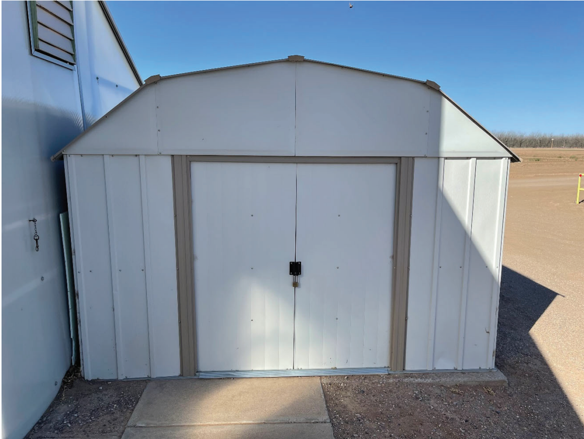
Metal storage shed: Needs: Gutter and down leaders.
