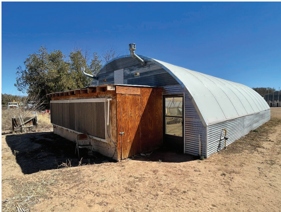
Green house plenum building, rotted wood. Building is beyond feasible repair if planning to continue use.
