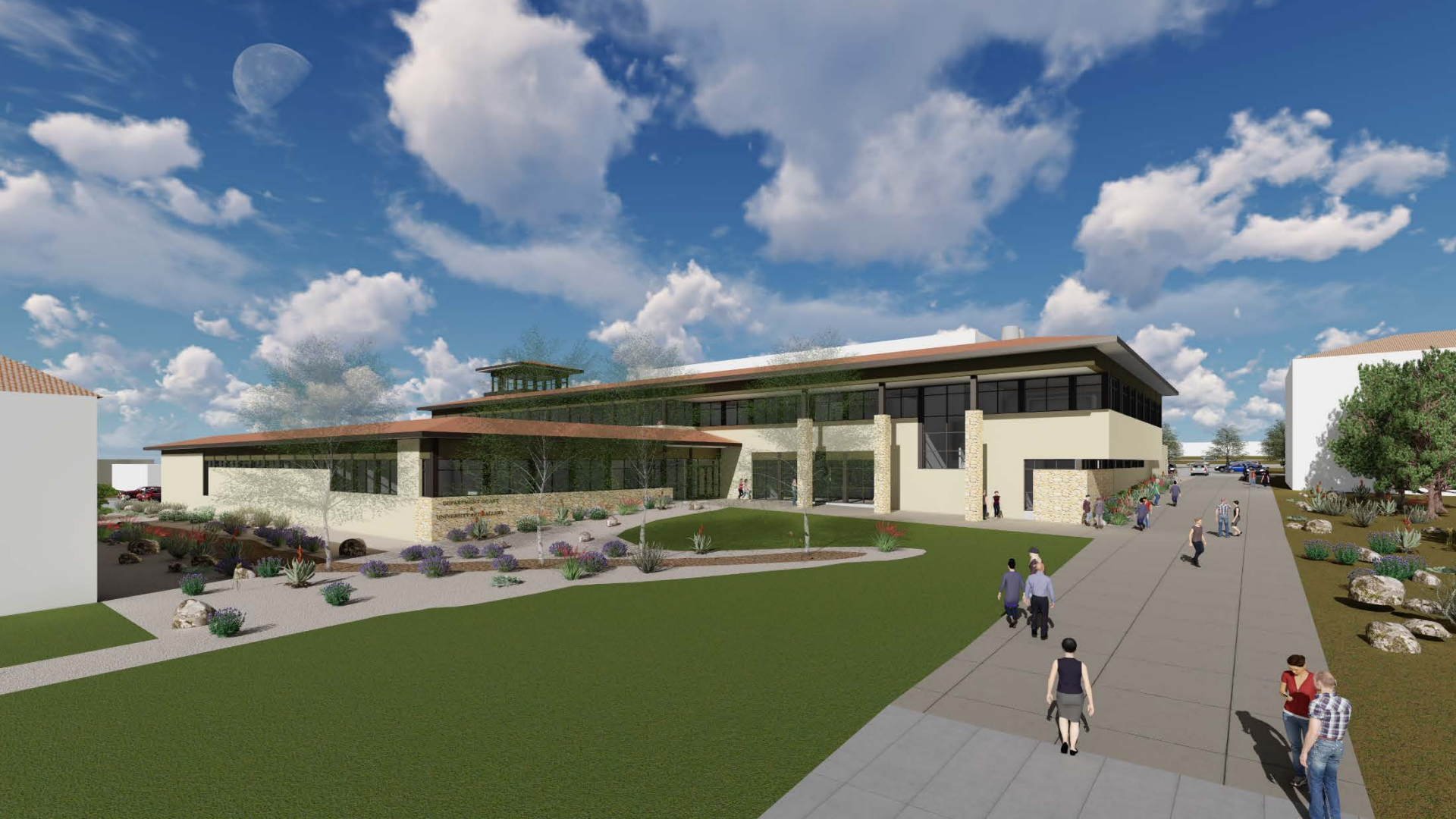
VIEW TOWARDS BUILDING'S SOUTHWEST CORNER
