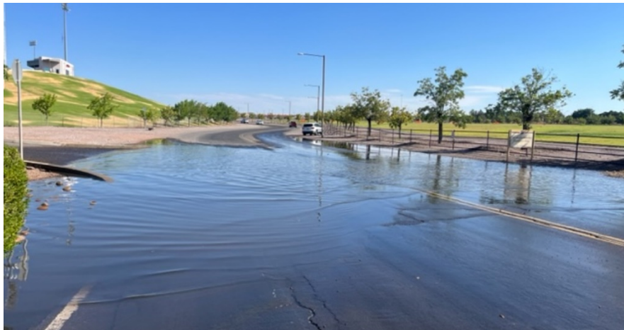
FIGURE 5-4: PONDING AT ARROWHEAD AND WELLS
