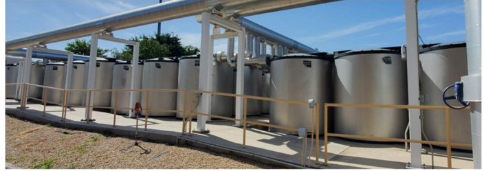
IMAGE 11 – SATELLITE PLANT ICE STORAGE TANKS
