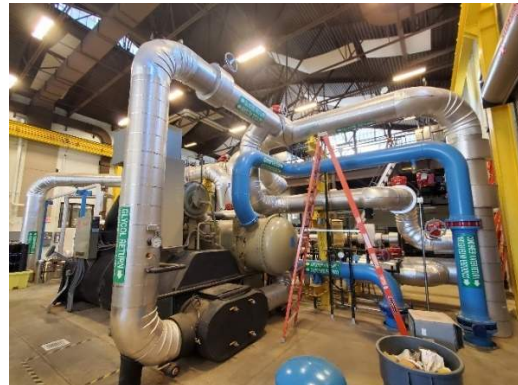
IMAGE 13 – SATELLITE PLANT CHILLER
