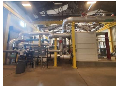
IMAGE 10 – SATELLITE PLANT ICE EXCHANGER
