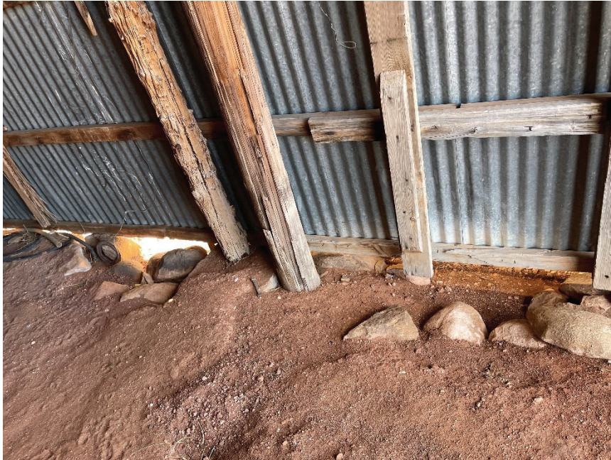
The single bay implement storage has rotted wood columns sitting on earth. It has erosion undermining foundation. Building beyond feasible repair
