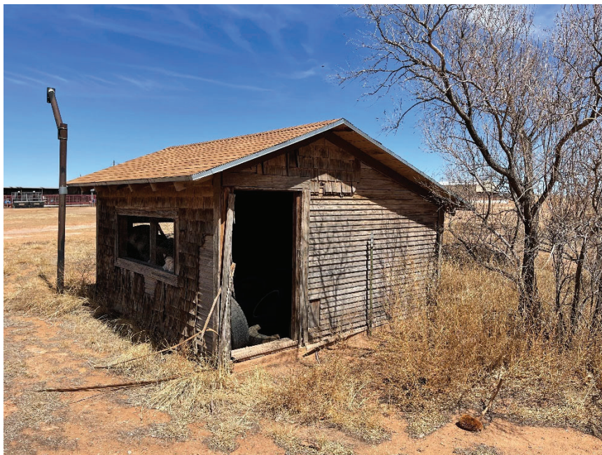
The tire storage is a combustible building with rotted wood throughout. Building beyond feasible repair
