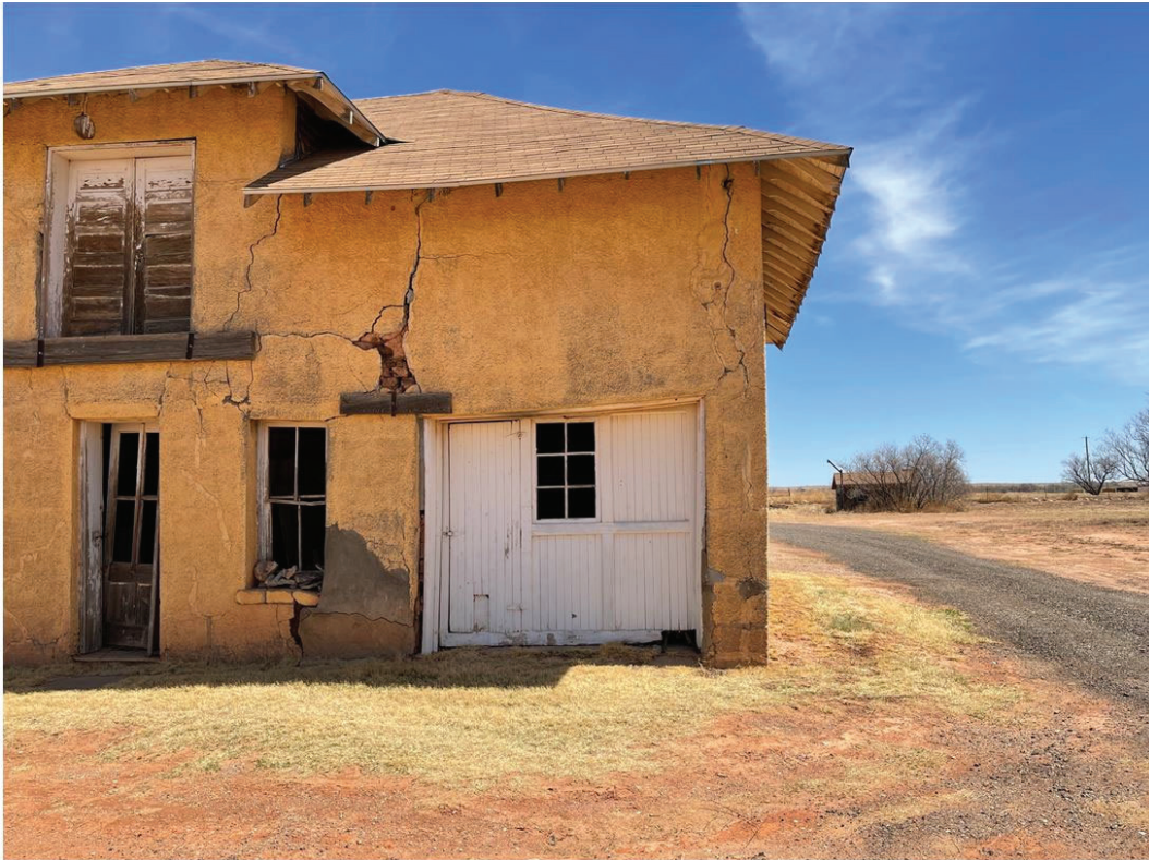
Close-up view of structural cracking and differential settlement. This condition is typical.
