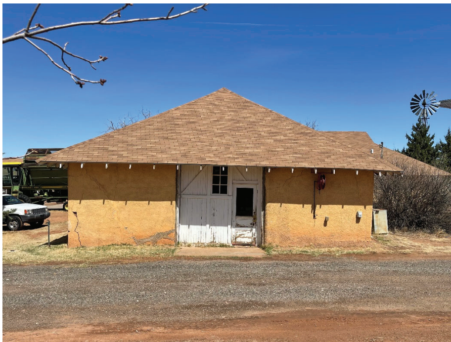
Shop building has differential settlement. Building is beyond feasible repair.
