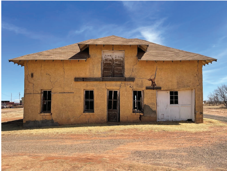
Horse barn has differential settlement. Building is beyond feasible repair.
