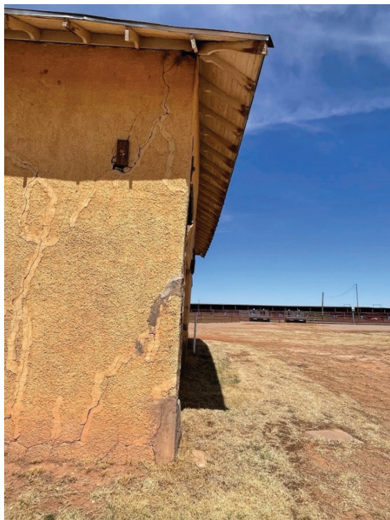
View of Southeast corner showing wall leaning out with differential settlement. This condition is typical.
