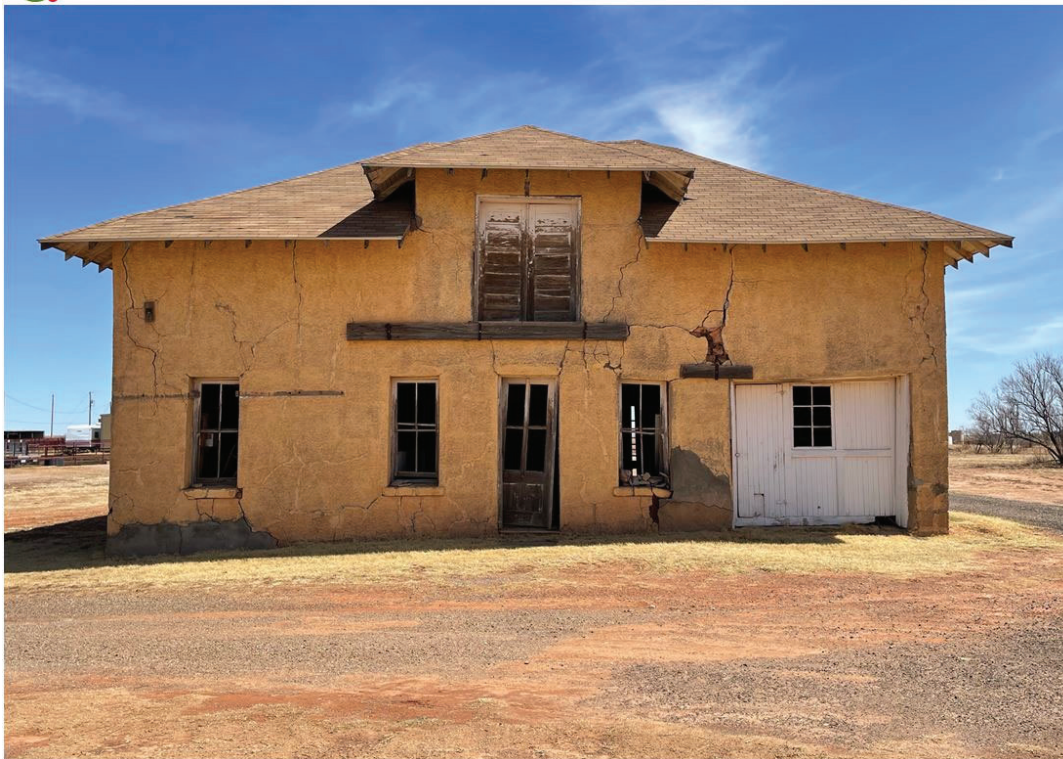
View of main façade showing structural cracks throughout the adobe walls due to differential settlement. This condition is typical.
