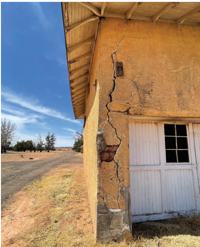
View of corner settlement and through-wall cracking. This condition is typical.
