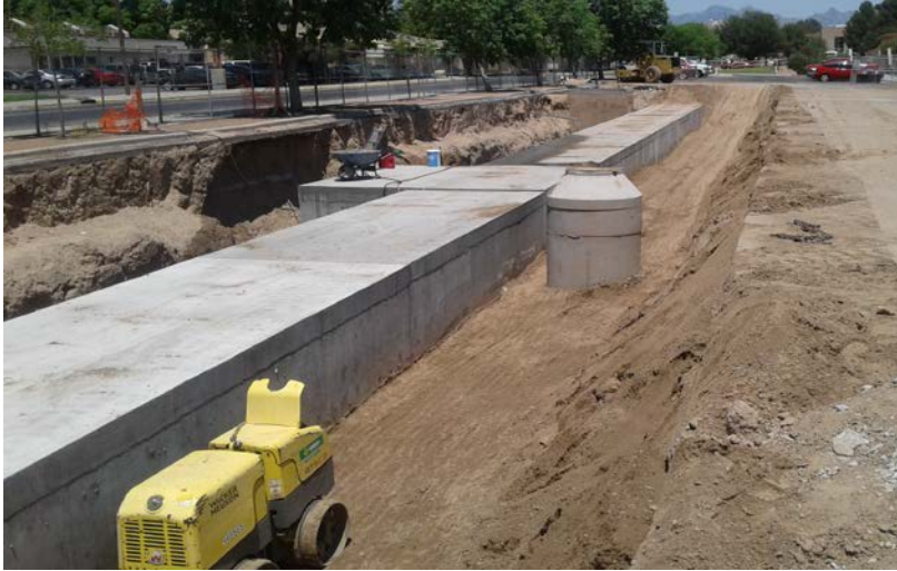
Phase III Repair 338 Lineal Feet Stewart St.
