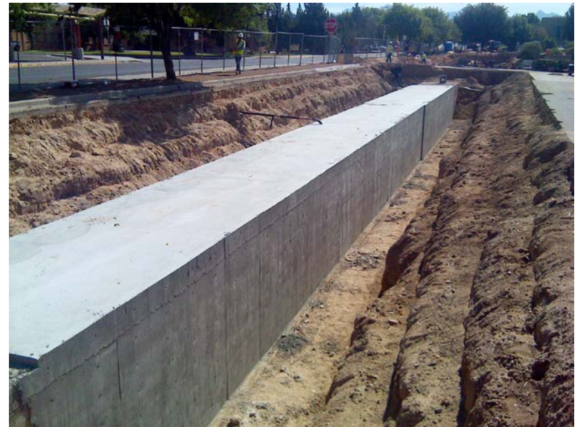
Phase I Repair 271 Lineal Feet Stewart St.
